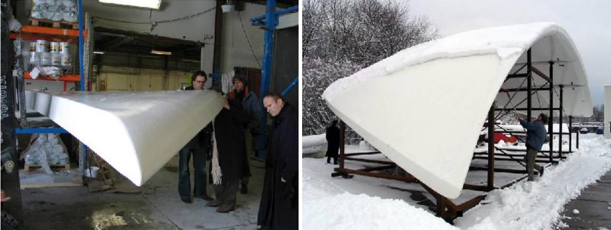
**Fig. 28-29. Roof segment (left) and fitting of all the roof segments of the lower wing of ‘The Library’ at Holland Composites in March 2005.**
