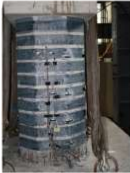
Figure 8. Column, strengthened by CFRP strips after the experiment
