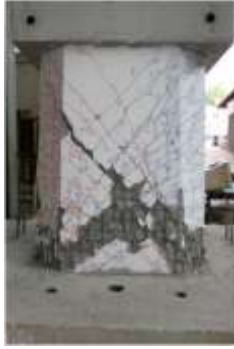
Figure 6. The investigated as-built column after the failure
